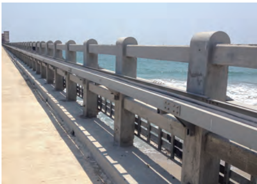
Chennai Refinery - Jetty - 2007
