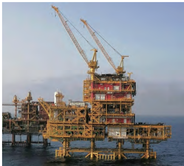
GRP cable ladder and trays on offshore
